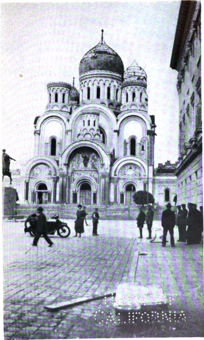
THE RUSSIAN CHURCH BEING DEMOLISHED BY THE POLES AT WARSAW.
